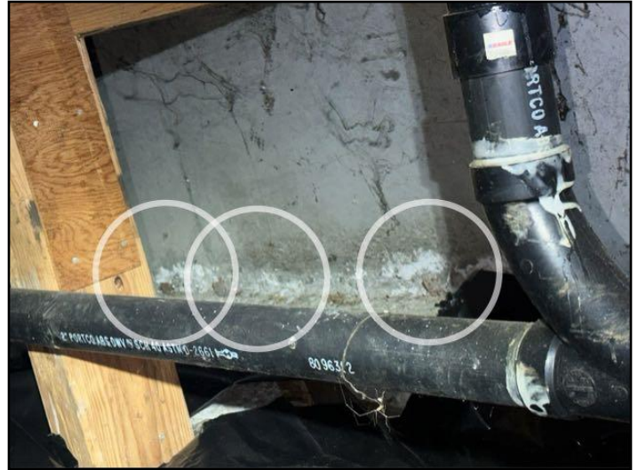
170. Efflorescence
