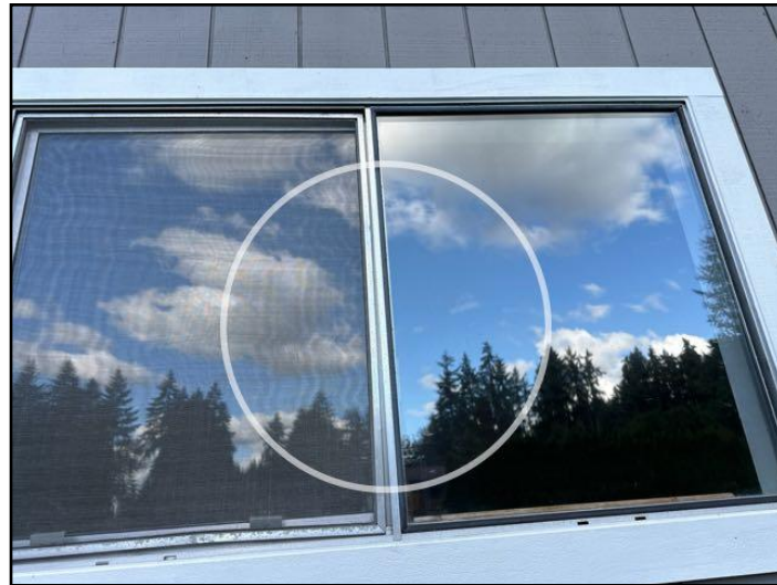
59. Lost seal on double or triple glazing
